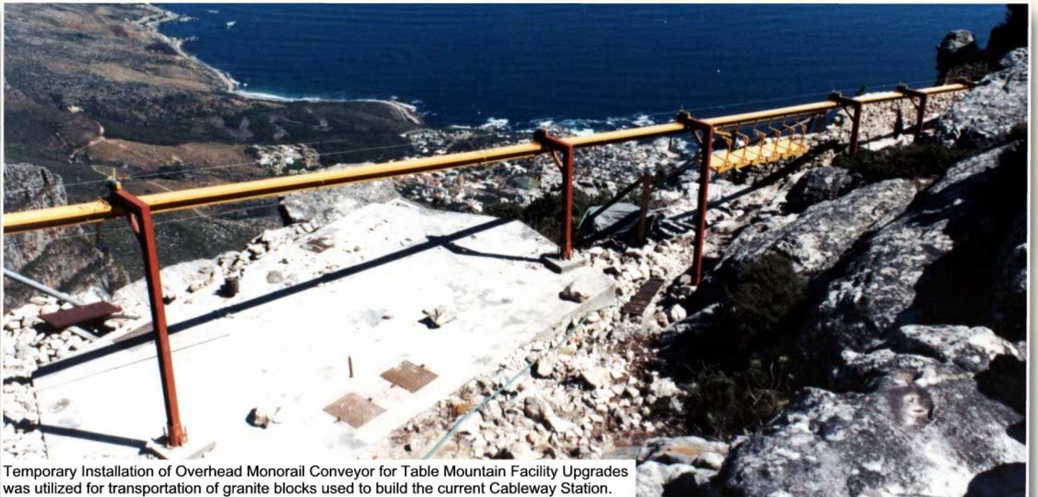
Temporary Installation of Overhead Monorail Conveyor for Table Mountain Facility Upgrades was utilized for transportation of granite blocks used to build the current Cableway Station.
